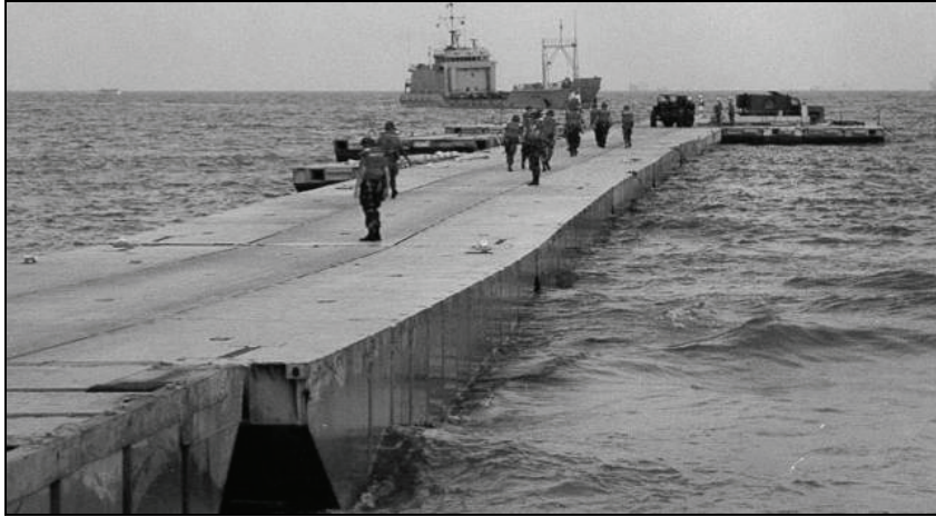
Figure 2-13. Modular Causeway System (Floating Causeway)
